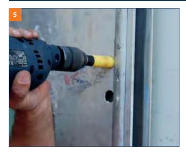
Make the holes from inside with a hole saw. Milling and eliminate any ridges or edges inside the counterbore in order to properly position and align the spacer. The inner holes of 20-22 mm accommodated the supplied spacers, which avoid the crushing of the sheet metal. Some grooves on the surface are provided to facilitate the cut and allow the padlock to adapt to different thicknesses of sheet metal and interspace.
