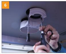
Secure the intermediate piece using the four screws.
